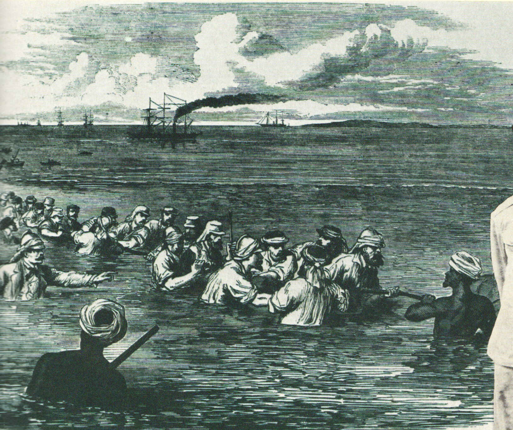
A cable is landed at Fao, on the Persian Gulf, in 1865. From here it crossed the Indian Ocean, providing the final link in a telegraph system joining Europe and India.
