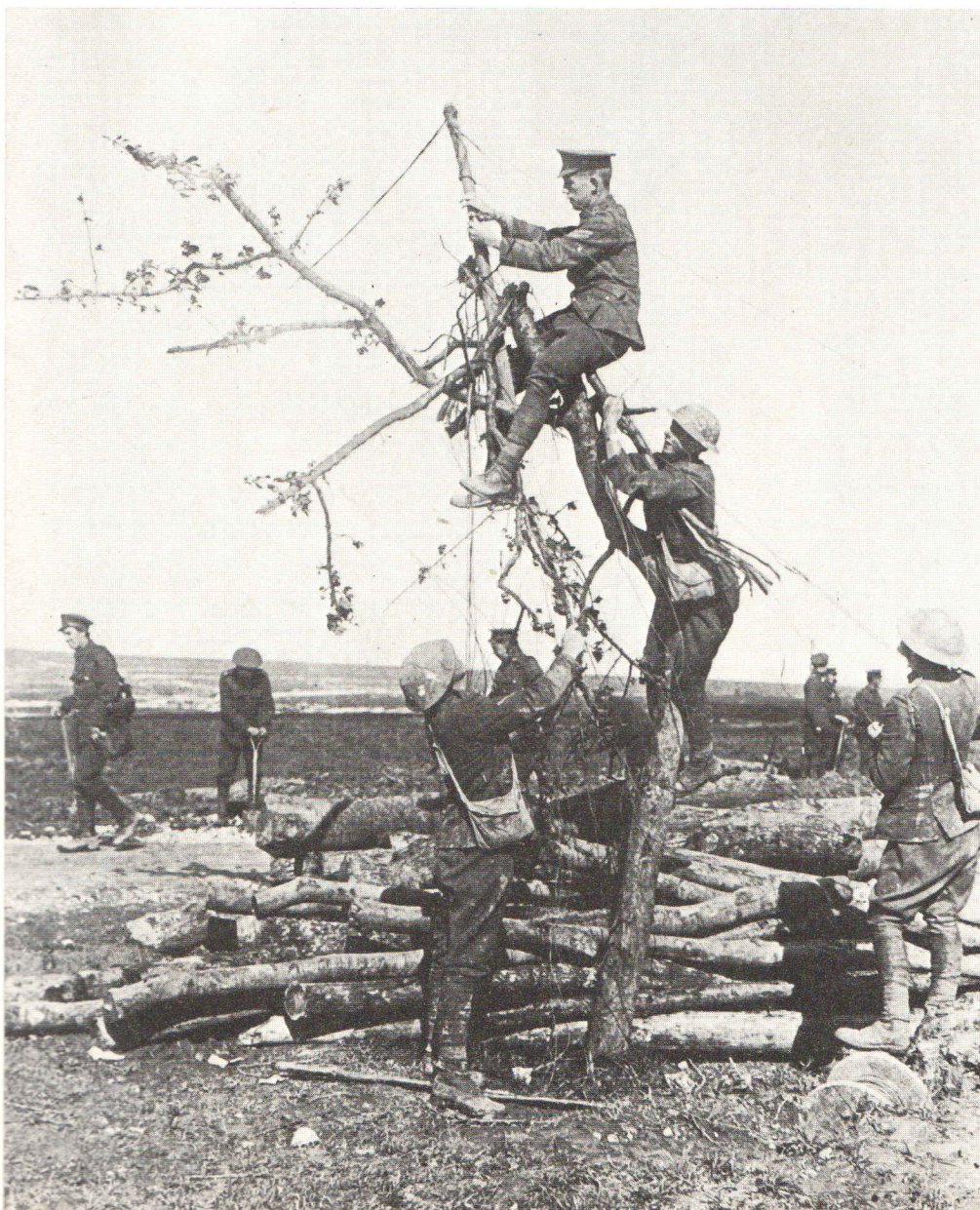
A telephone line is rigged up in a sector of the Western Front in 1916. Wires were often hit by shellfire, but mass attacks depended on the telephone for co-ordination.
